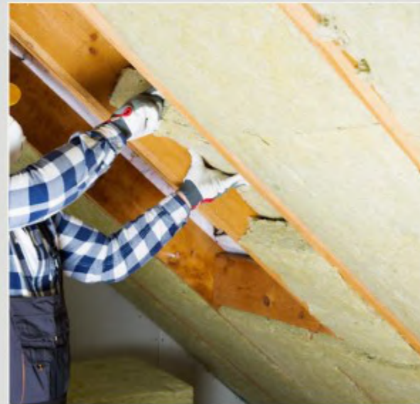
Roof Thermal Insulation
