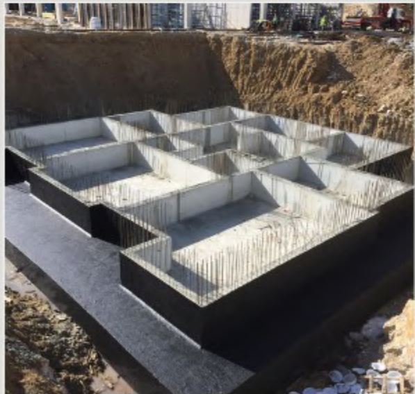
Foundation Hydro Isolation
